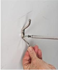
5. Secure one end of the rope to the cleat. Take the rope up the ladder and put it through the pulley hole. Hold onto this end of the rope as you descend the ladder.
