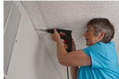
Screw the screw hooks into the holes. The screw hooks should angle slightly upward. Place each pulley swivel loop onto each hook.
